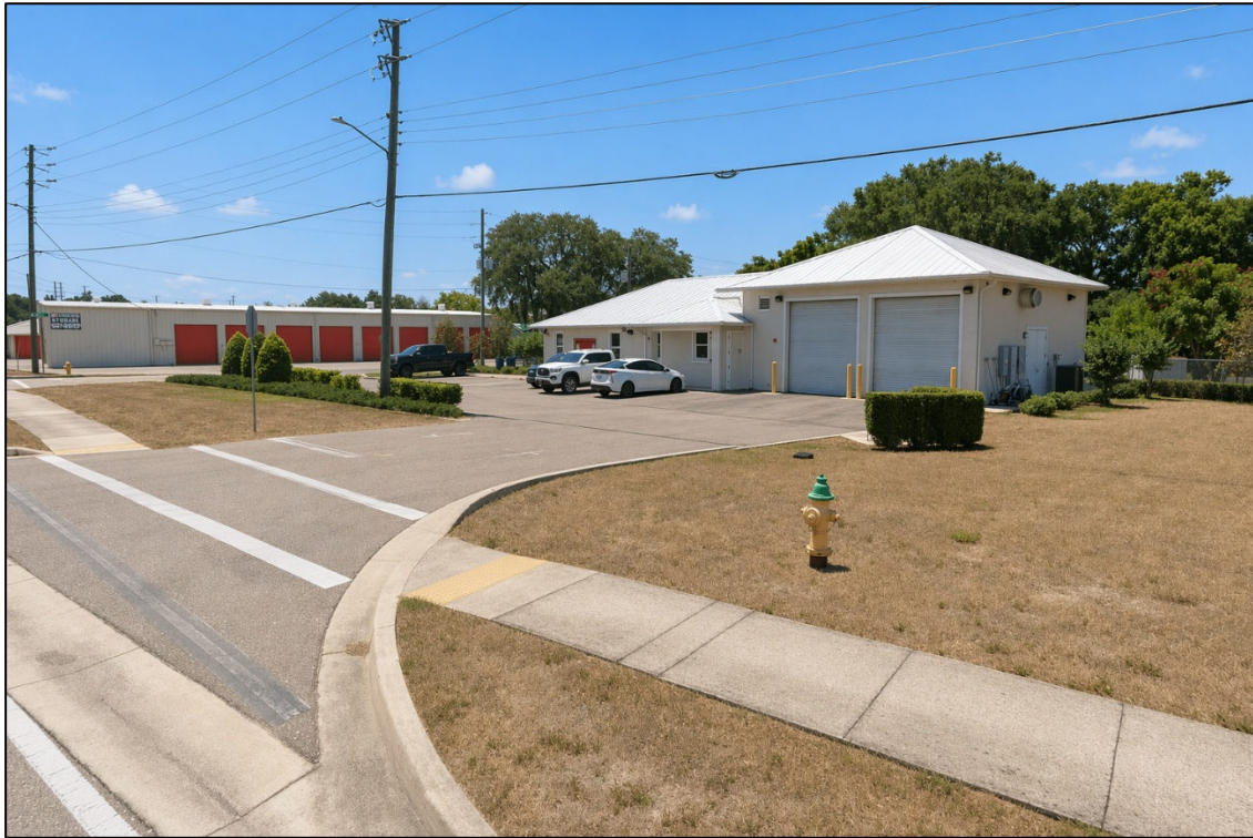
Figure 10: Existing Conditions of Highlands County Fire Rescue EMS #17
