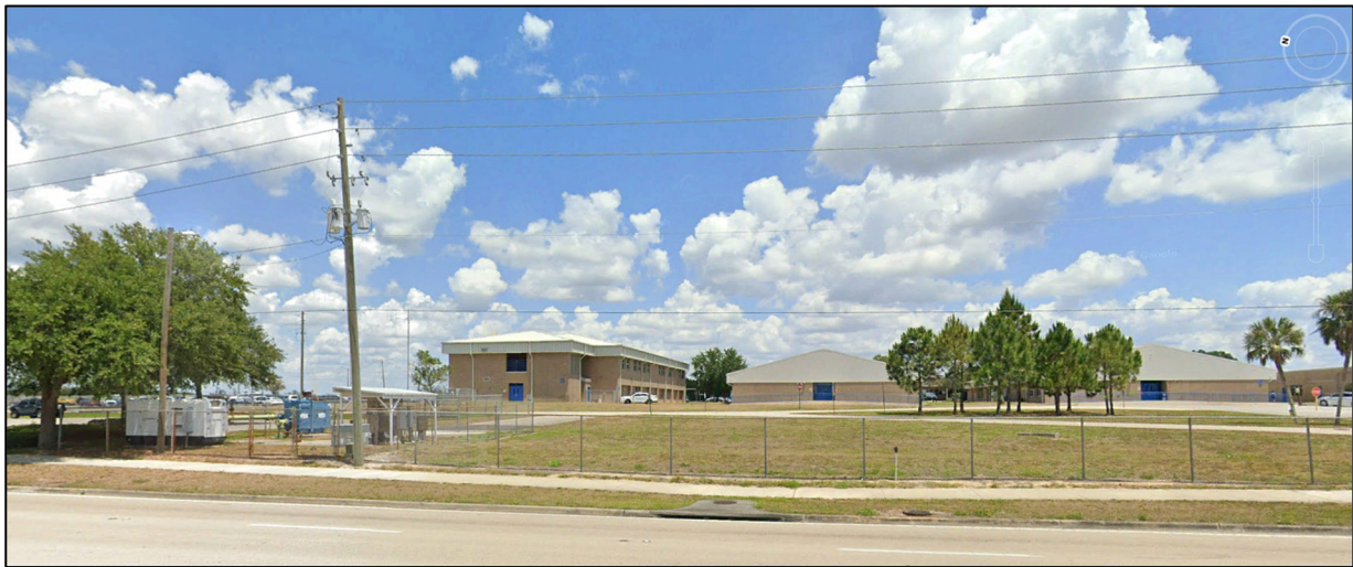
Figure 8: Existing Conditions of Sebring High School
