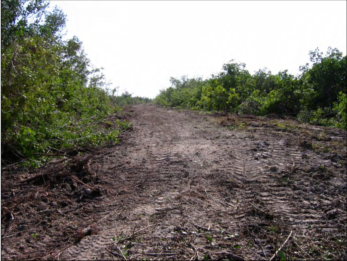
Figure 7: March 18, 2008 Completed fill of Large Ditch
