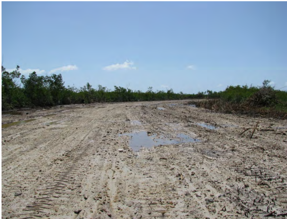
Figure 8: April 4, 2008 Completed Fill of Large Ditch
