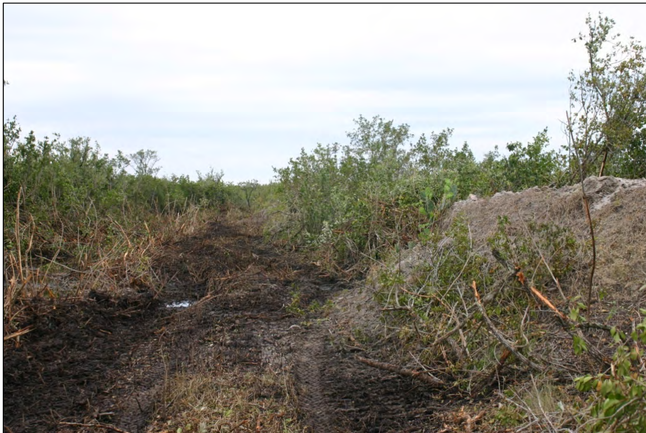
Figure 4: March 11, 2008 Ditch Restoration
