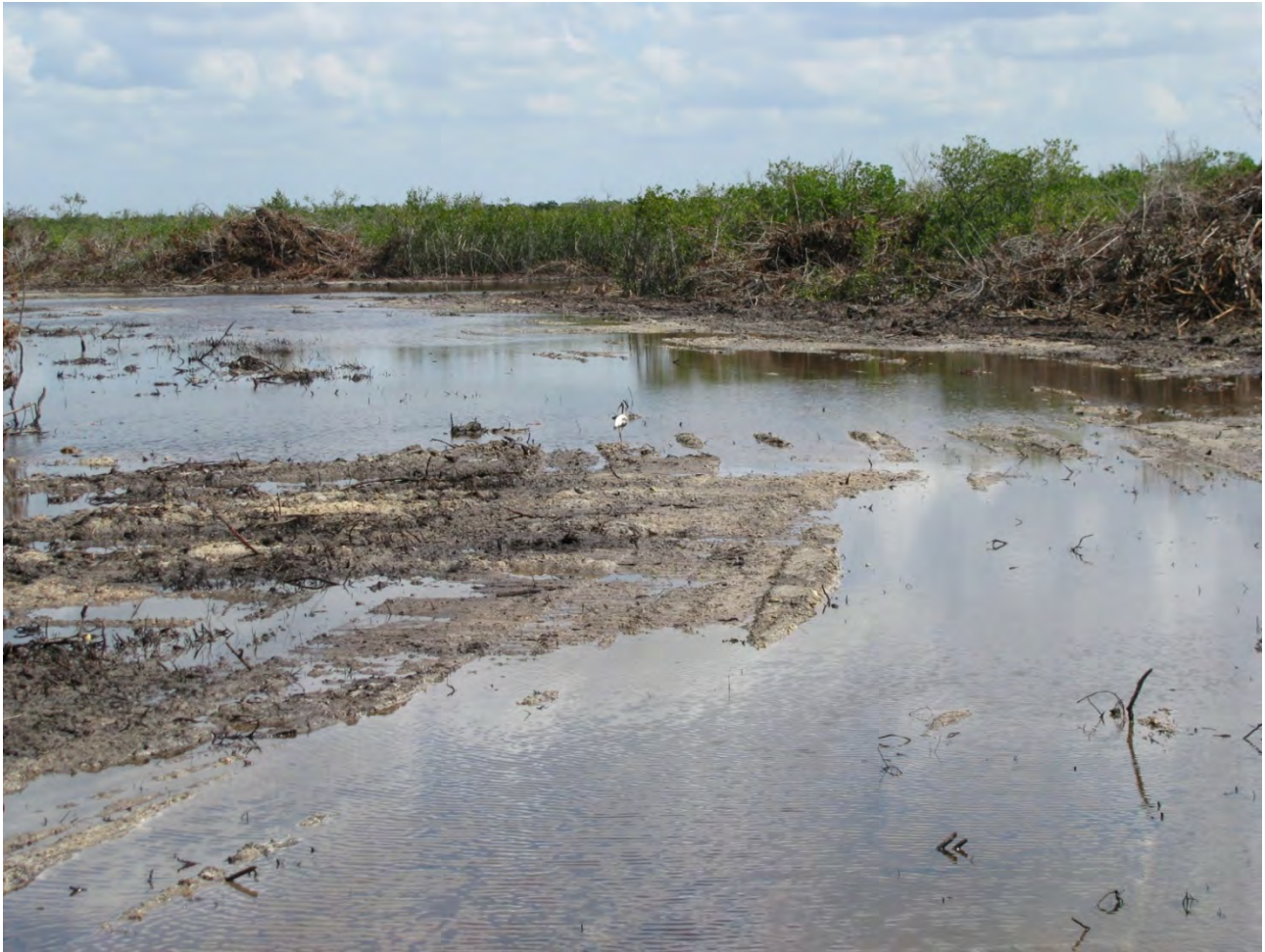
Figure 9: April 23, 2008 Flooded Works site for Heron.
