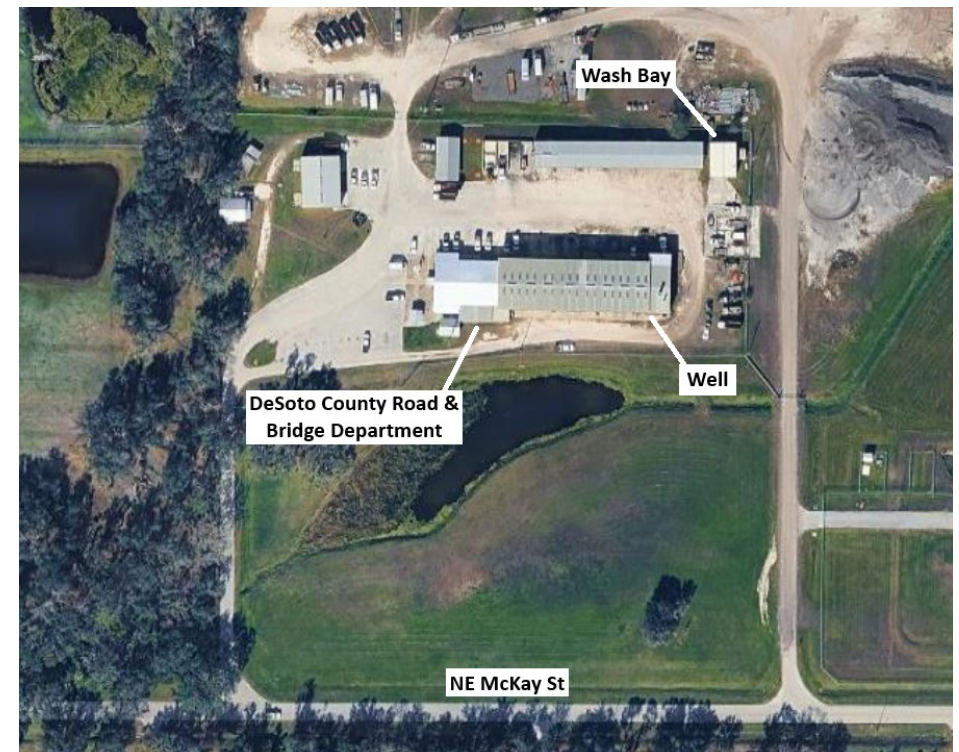
Figure 6: DeSoto County Road & Bridge Department, Wash Bay, and Well
