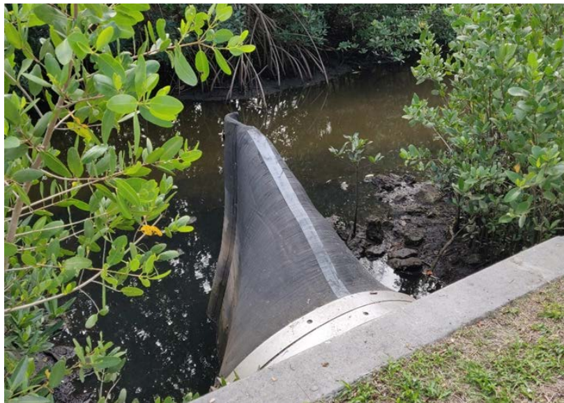
Photograph 4.2 Stormwater Check Valve for Backflow Prevention
