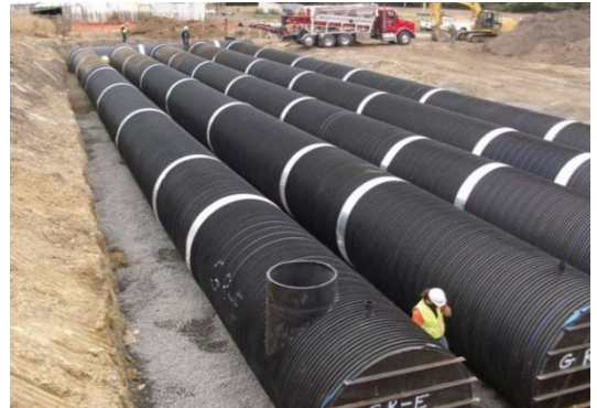
Storage Tanks for Excess Runoff ( www.conteches.com )
