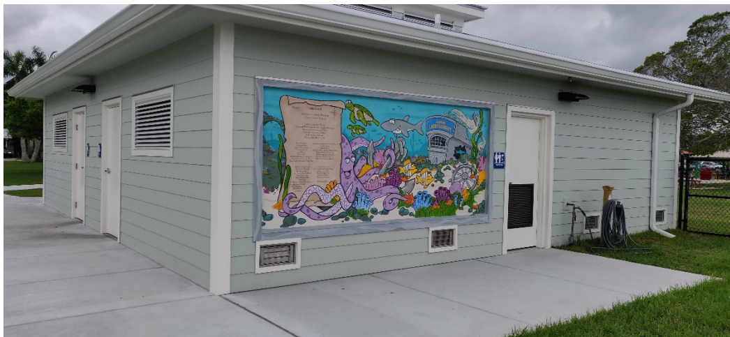
Photograph 4.4 Flood Vents for Wet Floodproofing at Gilchrist Park
