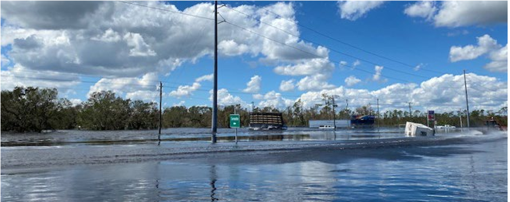
Figure 36: Flooding in DeSoto County during Hurricane Ian
