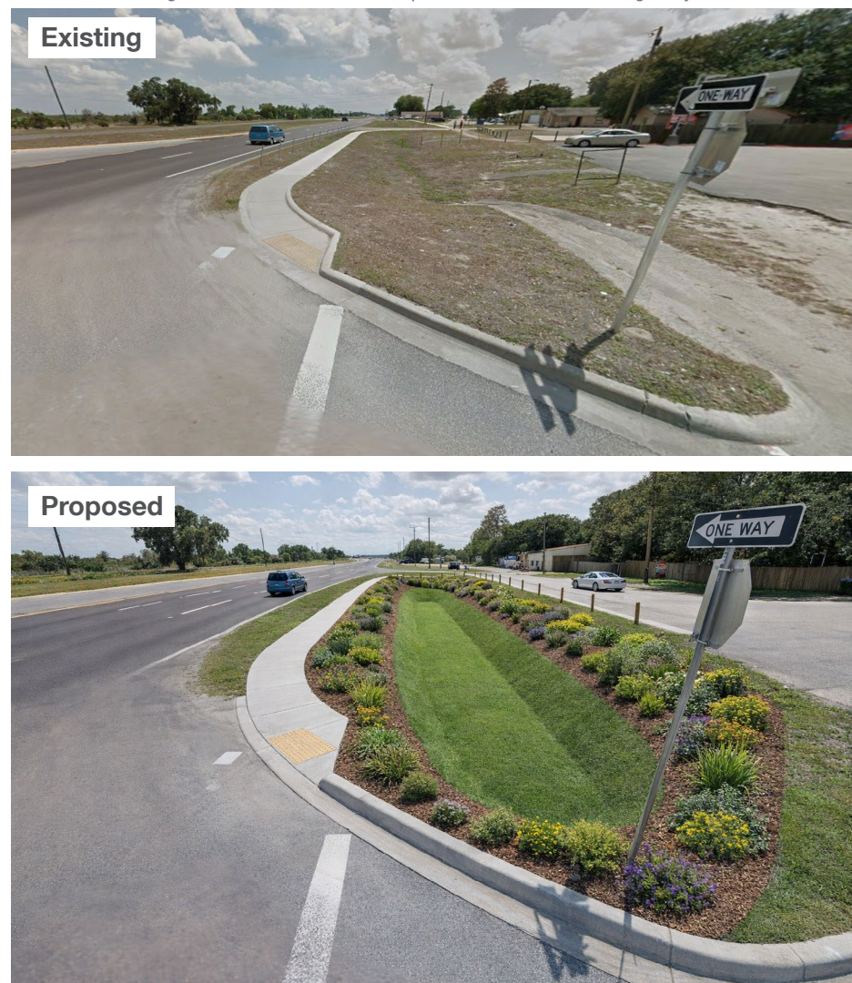
Figure 17: Visualization of Upsized Swales on US Highway 17
