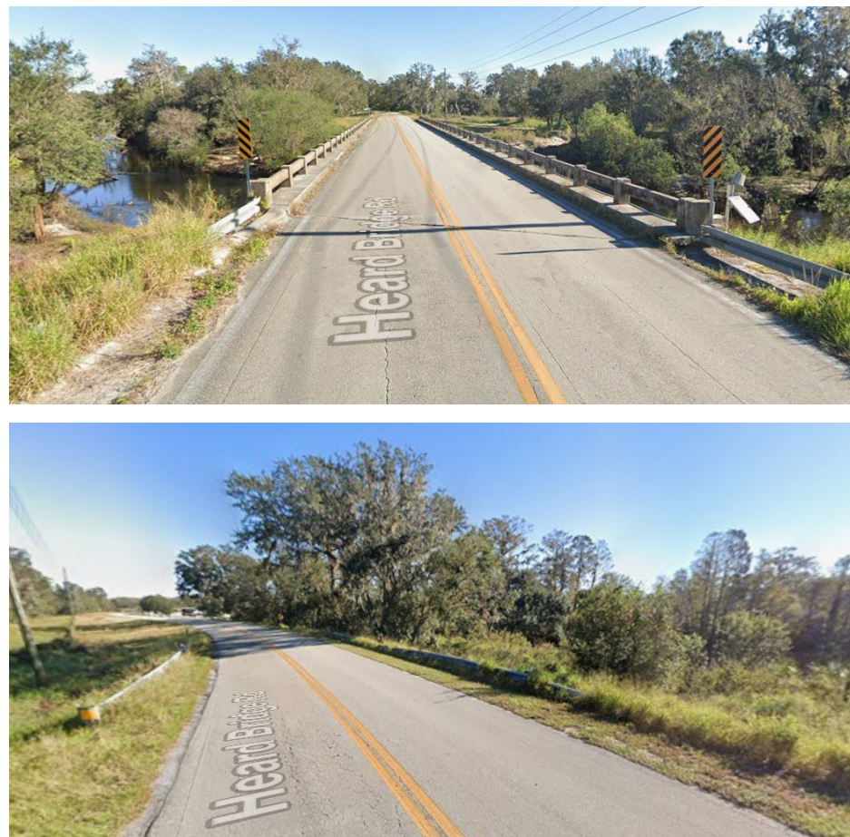
Figure 7: Heard Bridge Rd Bridge (Top) and the Heard Bridge Rd Culvert (Bottom)
