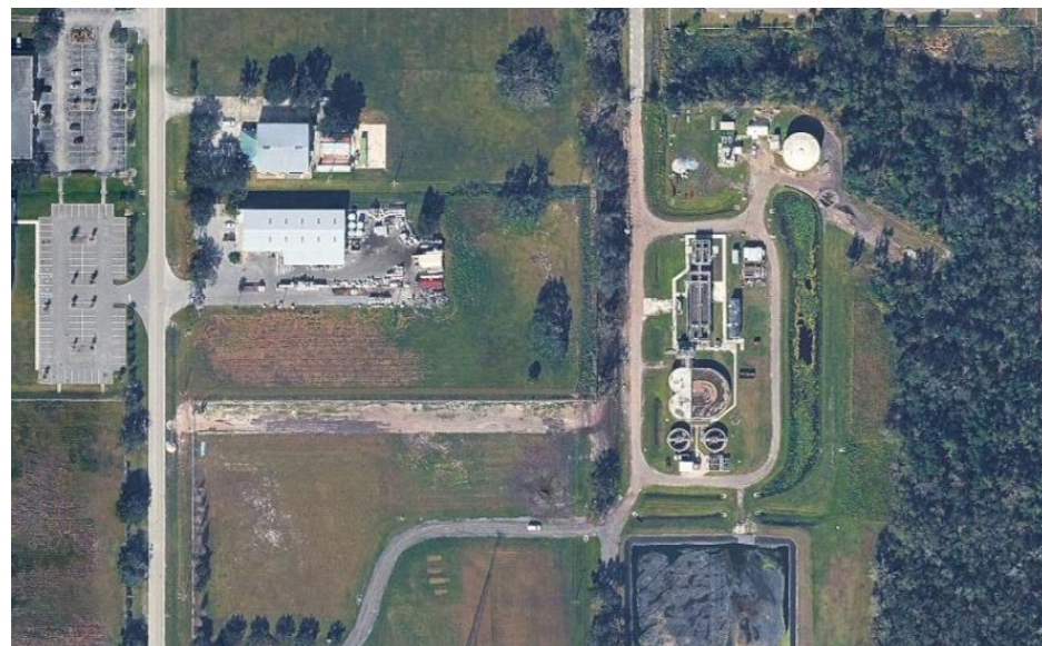
Figure 5: Wauchula Hills Water and Wastewater Treatment Facility
