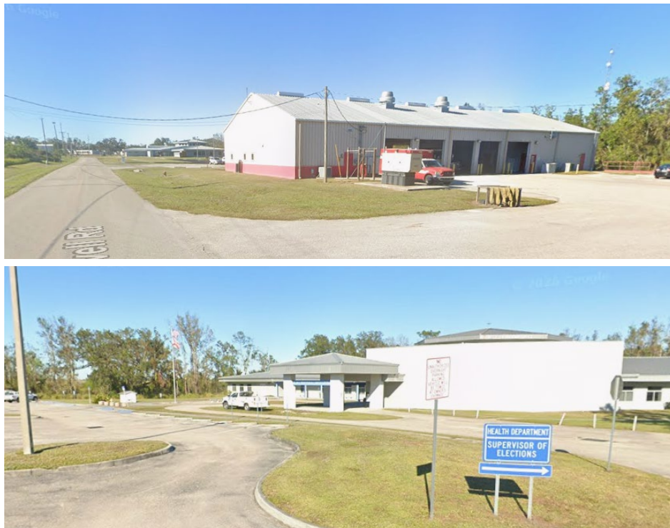
Figure 6: Hardee County Fire Rescue Administration (Top) and Hardee County Health Department (Bottom)
