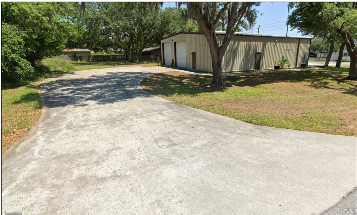
Figure 10: Existing Conditions of Highlands County Fire Rescue EMS #18
