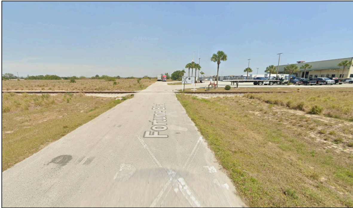
Figure 8: Existing Conditions at Railroad Crossing at Fortune Boulevard
