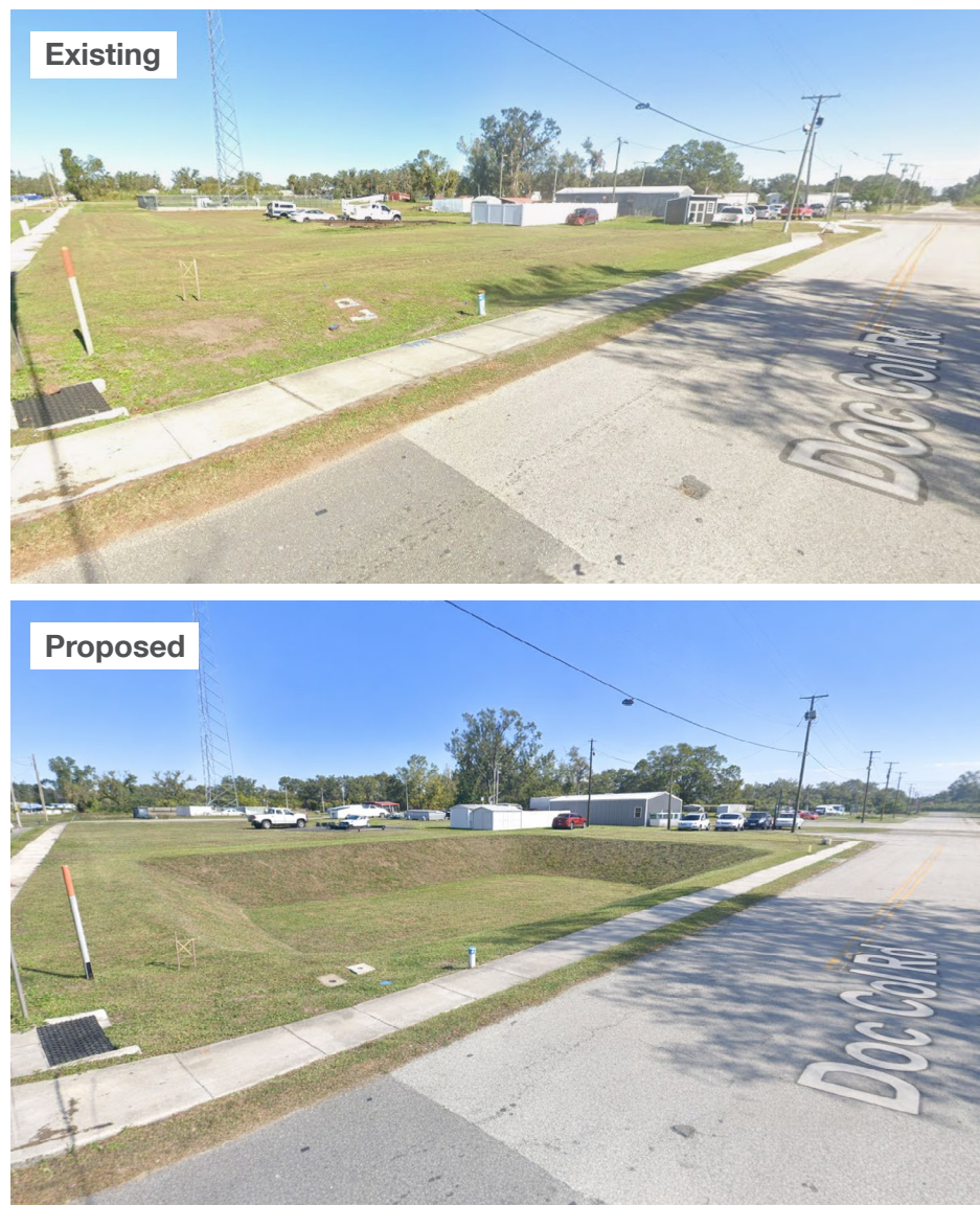
Figure 15: Visualization of Roadside Swale along Doc Coil Rd
