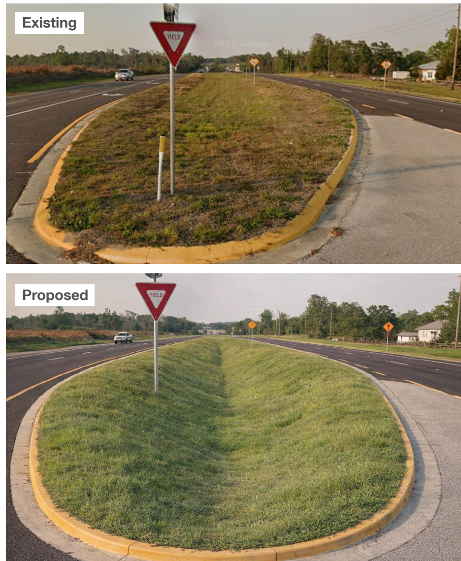
Figure 14: Visualization of Upsized Swale in the Median of US Highway 17 Located at the Evacuation Route Segment
