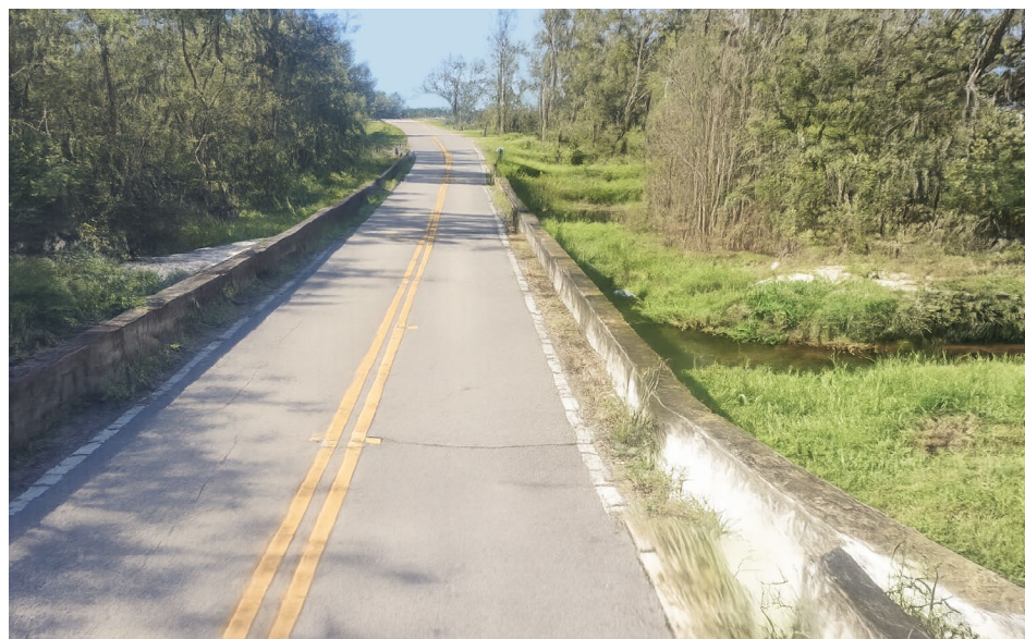
Figure 5: Country Rd 664 Bridge Crossing Little Payne Creek
