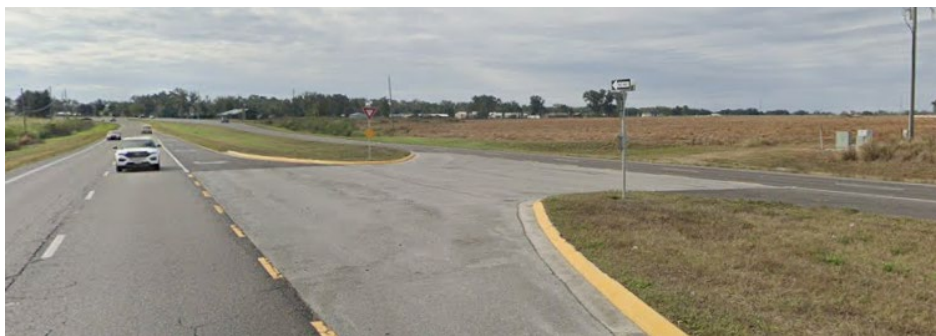
Figure 7: Turn lane prone to flooding on US Highway 17
