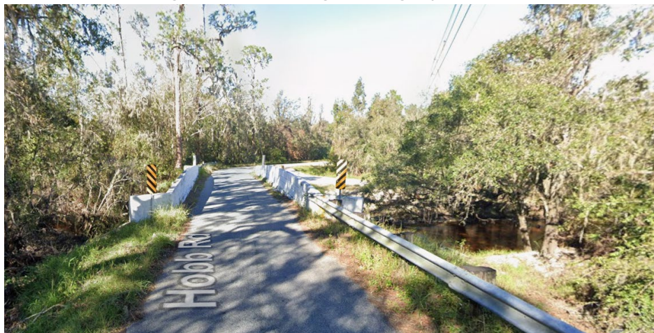
Figure 6: Hobb Rd Bridge Crossing Payne Creek
