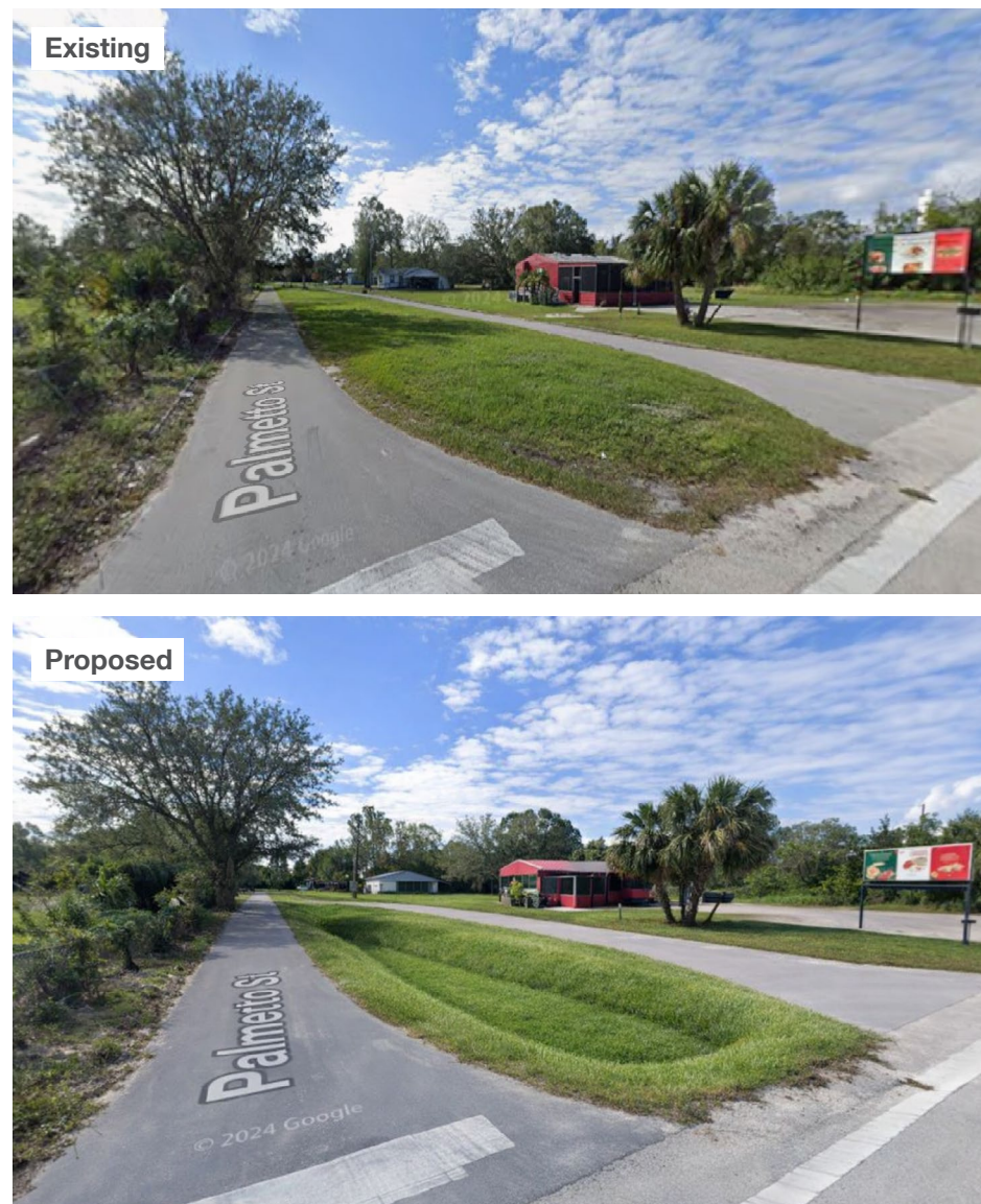
Figure 15: Visualization of Roadside Swale at the Evacuation Route intersection of Palmetto St and State Rd 66
