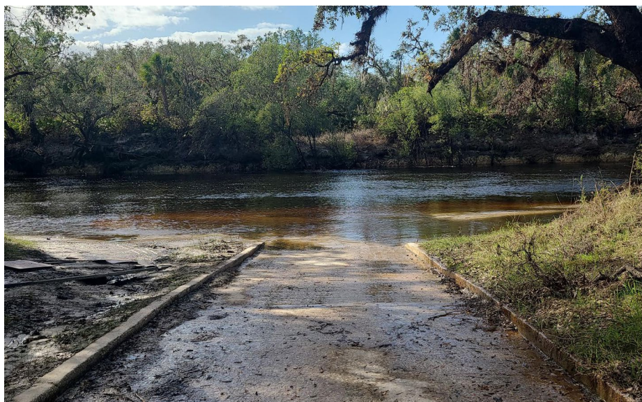
Figure 9: Flooded roadway along River Road SW, Zolfo Springs
