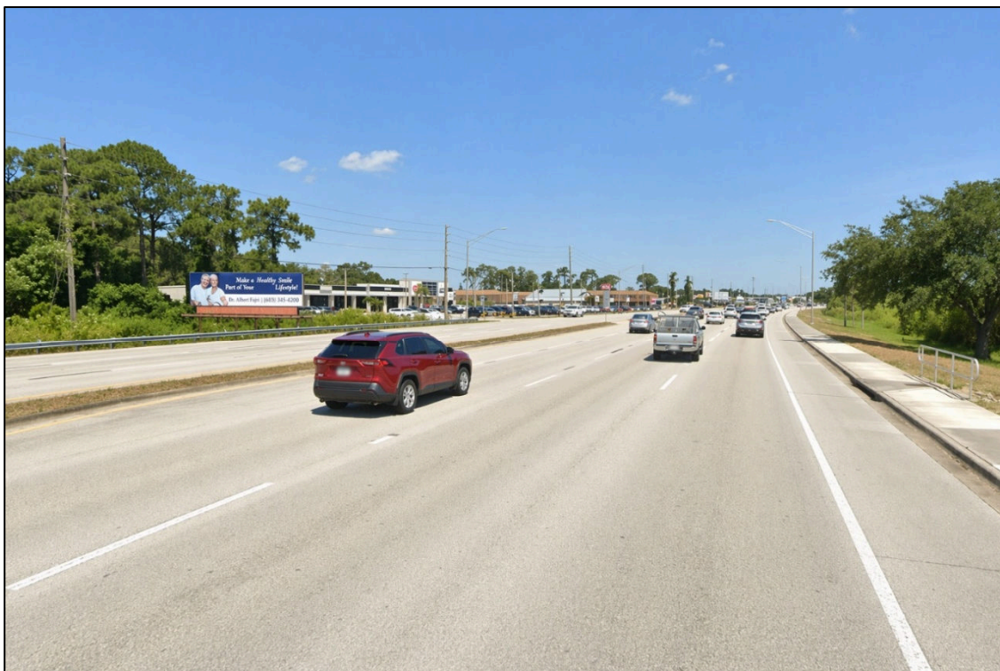
Figure 12: Existing Conditions of Highway 27 S
