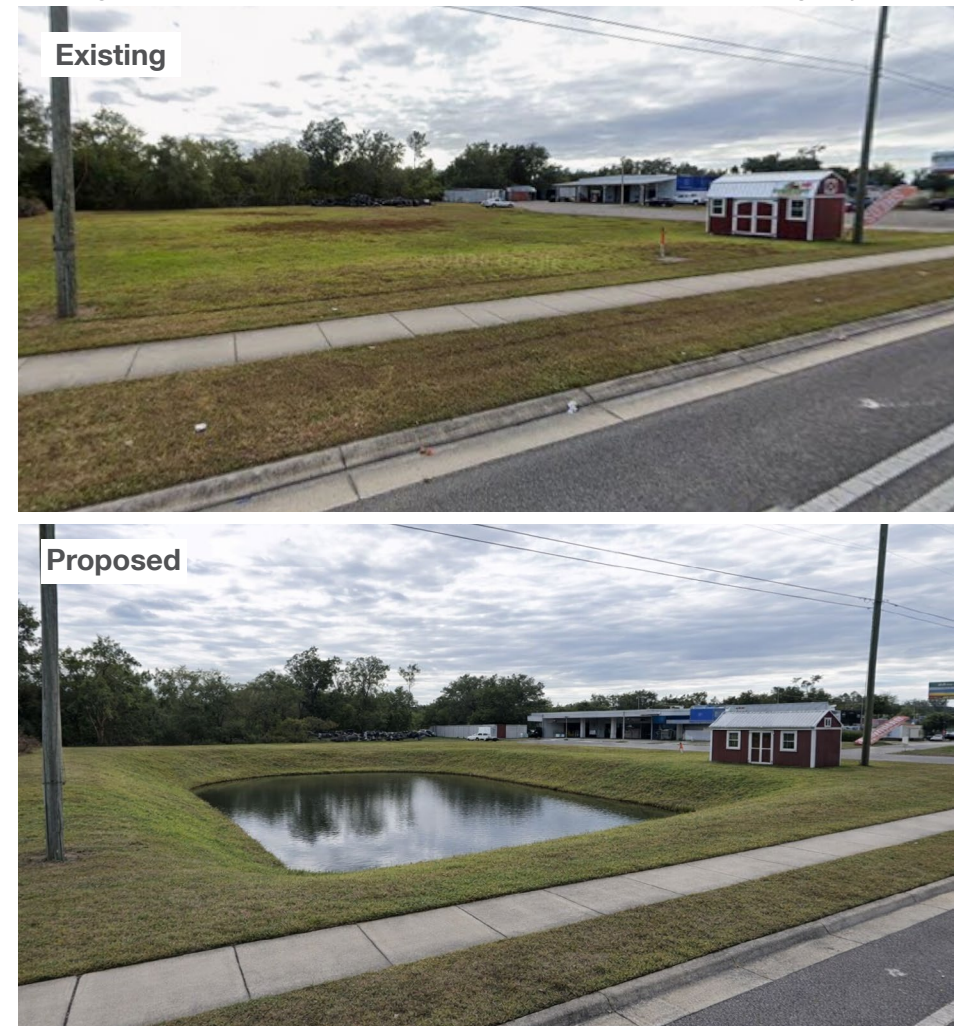
Figure 17: Visualization of Detention Pond at Price Child St and SW Highway 17
