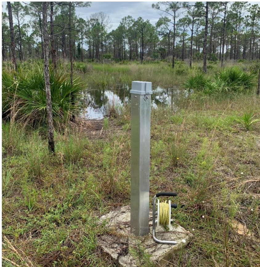
Figure 2-3. Groundwater Monitoring Station BW-11, August 2021
