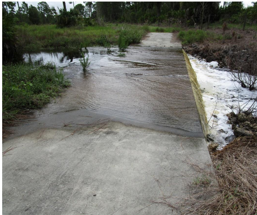
Figure 3-17. Concrete Low-water ford in South Yucca Pens
