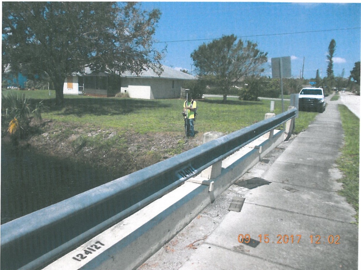
West side of bridge
