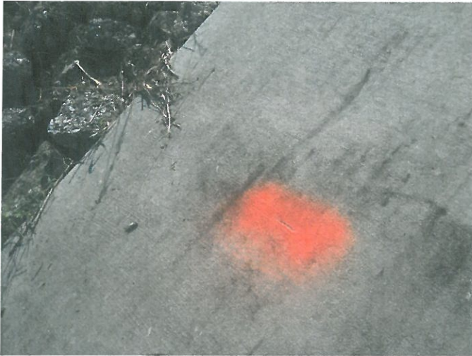
South side of weir
