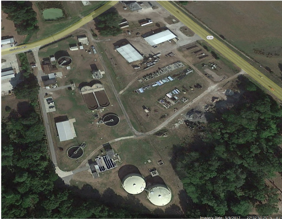
Example: Wauchula Wastewater Treatment Plant 2017 Google Earth
