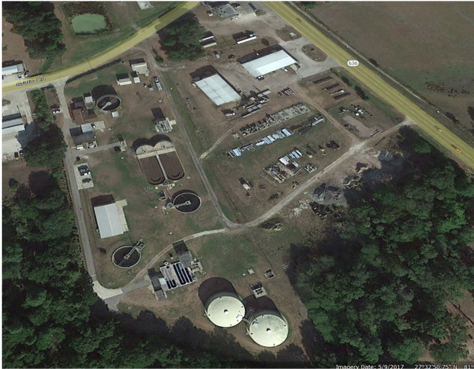
Example: Wauchula Wastewater Treatment Plant 2017 Google Earth
