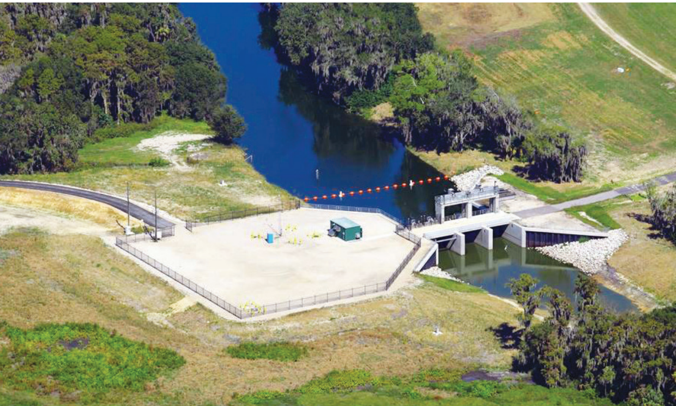
▲ Figure 22. SWFWMD completed replacement of Structure P-11 at the outfall from Lake Hancock in 2013. The new structure increases storage in the lake to provide increased flow downstream to the Peace River in the dry season | SWFWMD.
