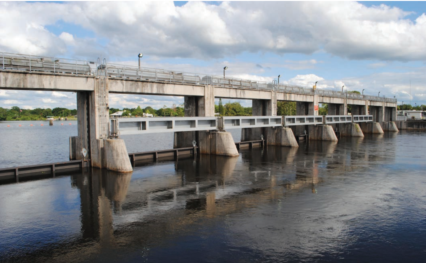
▲ The W.P. Franklin Lock and Dam on the Caloosahatchee River near Fort Myers was constructed to store water for irrigation and navigation. The dam starves the downstream Caloosahatchee Estuary of freshwater during dry periods and floods it with too much freshwater during the wet season | USACE.
